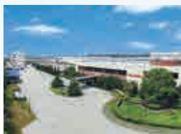
China Plant (MCC)
